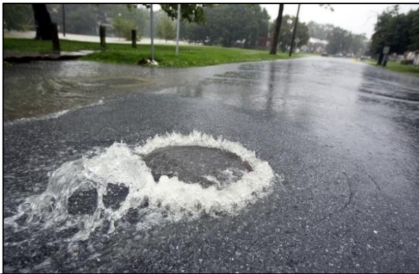
Figure 9: An example of typical highway and sewer flooding
