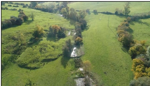
Figure 18: Aerial view of a few of the many Natural Flood Management features installed as part of the 3-year Defra pilot project. We have submitted a business case for this to continue for the next six years
